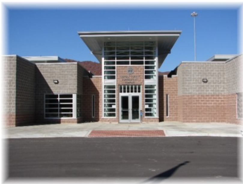
2009—Morgan County Correctional Complex
