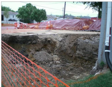
Excavation at a former drycleaner facility in Williamson County
