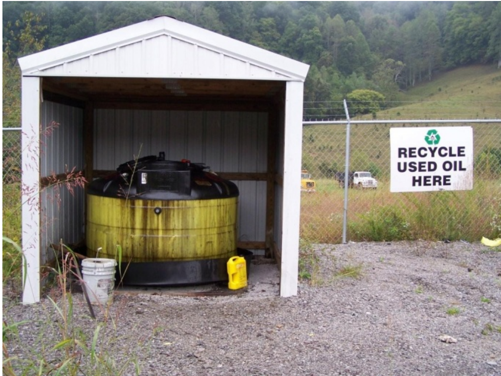
Figure 3: Used Oil Collection Tank at Hancock Convenience Center
