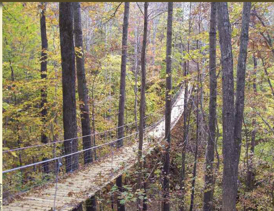
The second suspension bridge on Tims Ford State Park's newly completed Lost Creek Overlook Trail is 180 feet long. It traverses through the canopy of trees providing a view of surrounding trees and the forest floor below.
